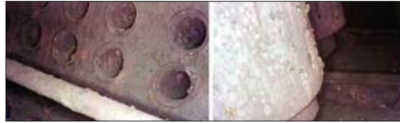
This image shows oxygen pitting in a boiler drum that was given inadequate layup protection. Courtesy: EPRI
